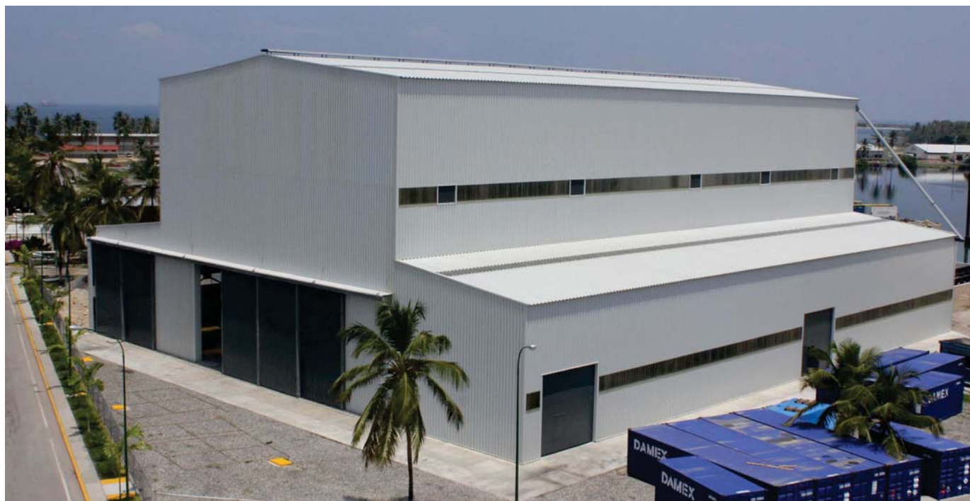
BACKSIDE OF THE PRODUCTION SHED
